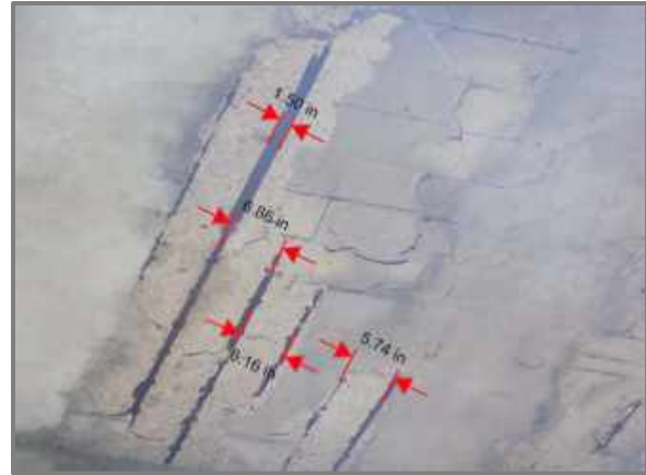
Photo 1 – Underside of deck spall from field investigation. Note that scaled dimensions from this photograph indicate a transverse rebar spacing much closer than 18".
