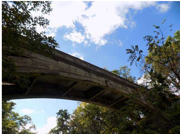
Photo 1: Lake Park Arch Bridge
