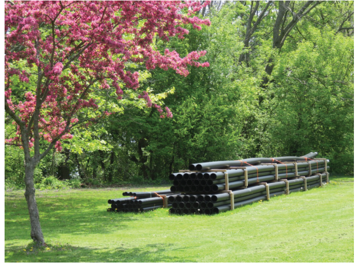
Irrigation piping is temporarily stored near the golf course storage shed.
